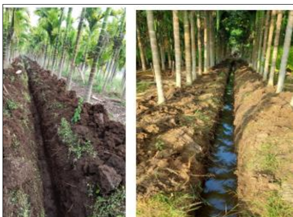
Fig 10: Demonstration of Open Drainage in Undrained Soils
